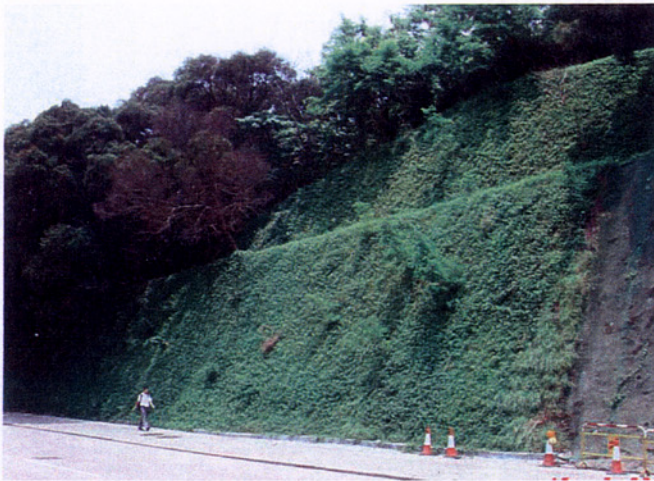
Overall view of slope treated with Rocksgrass
