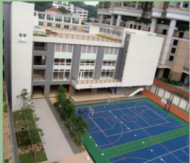
The project comprises the construction of a 6-storey 24-classroom school building consisting of a classroom block and an assembly hall block overall T-shaped on plan together with associated facilities.
