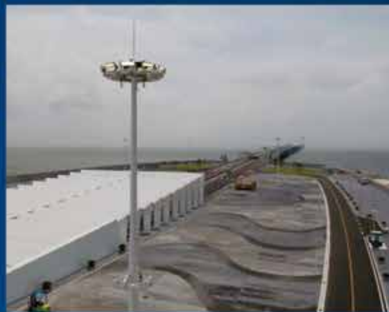
HK-ZHUHAI-MACAO BRIDGE - ARTIFICIAL ISLAND
