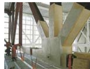
Fire protection for structural steel beam 鋼結構梁柱保護
