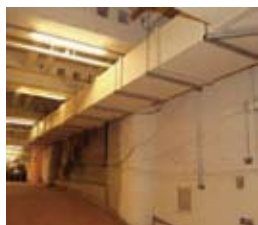
Fire-rated ducting 隔熱防火風管
