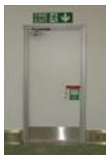
Fire-rated doors 隔熱防火門
