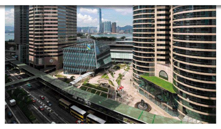
The Forum is an iconic gem in the middle of Hongkong Land's Exchange Square prime rental stronghold. The design of the five-storey office building adopts a simple and compact footprint of a box and redefines a well-connected outdoor public plaza. The building geometry was tilted by 15 degrees off one corner to open up a pleasant covered walkway across the site, allow for an elegant
