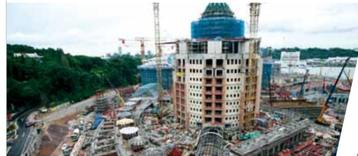
Construction began with the excavation of soil to construct the raft foundation, basement structures and support columns. A ground-level Environmental Deck, or E Deck, was cast above the basements. Made of reinforced concrete measuring more than a metre, E Deck supports the resort's hotels, attractions and landscape features that give the resort a lush, tropical look – hence its name. Four tunnels connect the basement to the surface road network and a new bridge built by Resorts World.
