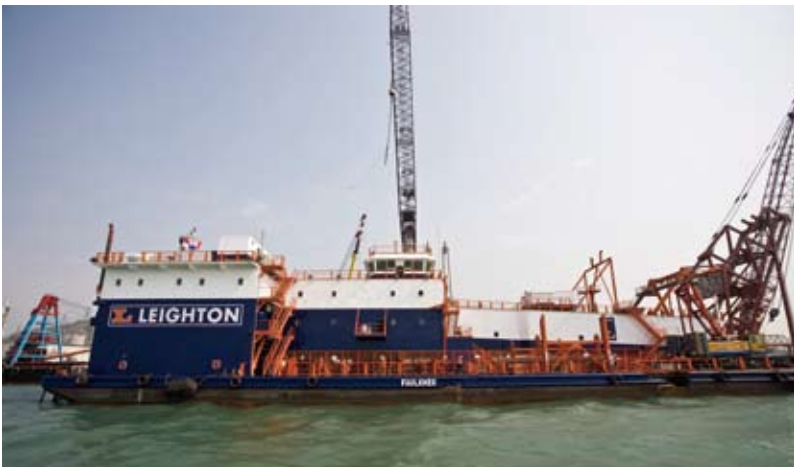
Leighton Faulkner at Permanent Aviation Fuel Facility project
