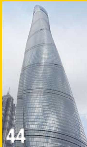
Shanghai Tower, Shanghai
