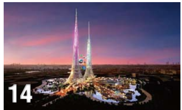
14 Phoenix Towers, Wuhan
